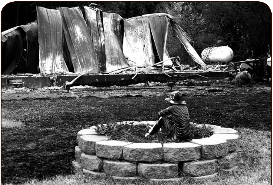
Fires have been all too common in Washington this year. Above is what was left of Lee and Lorna Barnhart's vacation home after the recent Cle Elum area fire. Lee reported that they hope to have it rebuilt by Thanksgiving.
