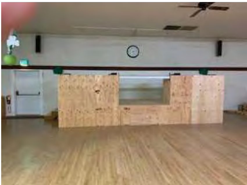
New stage under construction
