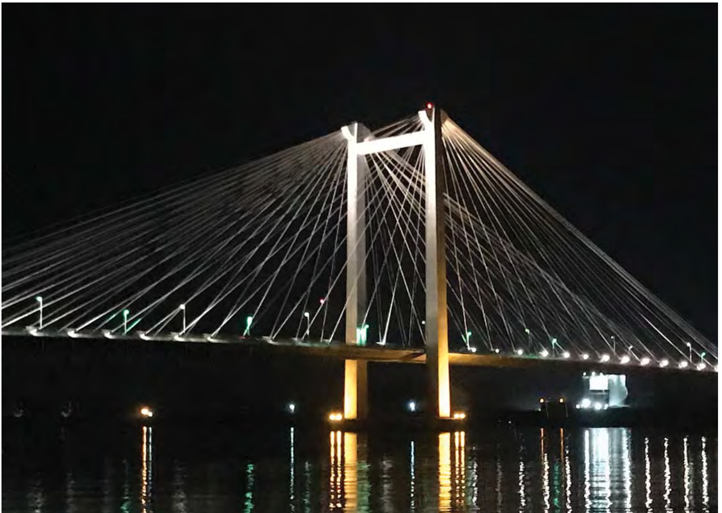
Cable Bridge on the Columbia River, Kennewick WA. Photo by Cynda Clark
